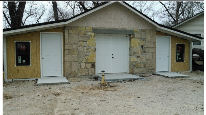
East elevation walls with windows and doors close in the stone shed wings
